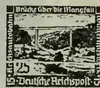
Bridge over the Mangfall SP84
