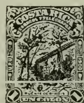
Birris Bridge A36
