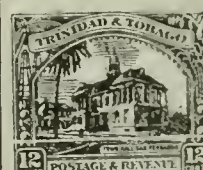
Town Hall, San Fernando A9
