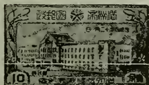
Postal Administration Building A26
