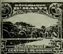
Aqueduct at Prince A53
