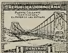
San Rafael Bridge A40
