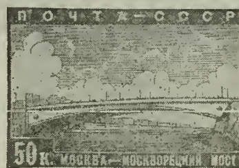
Bridge over Moskva River A313
