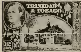
Town Hall, San Fernando A19
