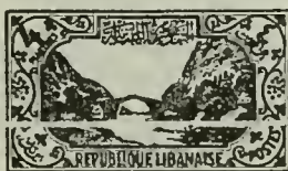
Bridge at Nahr-el-Kelb A13
