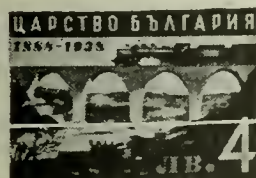
Train Crossing Bridge A162
