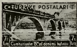
Railway Bridge A99
