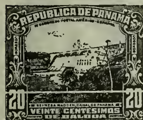
Madden Dam, Panama Canal A73
