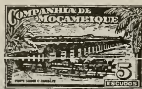
Zambezi Railroad Bridge A52
