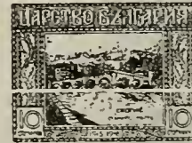
Bridge over Vardar River A56
