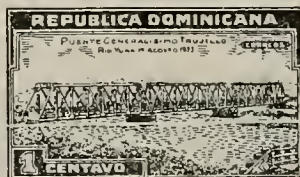
Trujillo Bridge A41
