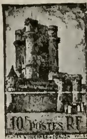
Turret and Gate of Vincennes A85
