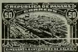
Drydock at Balboa A25
