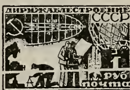
Constructing an Airship AP9
