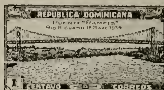
Ramfis Bridge A42
